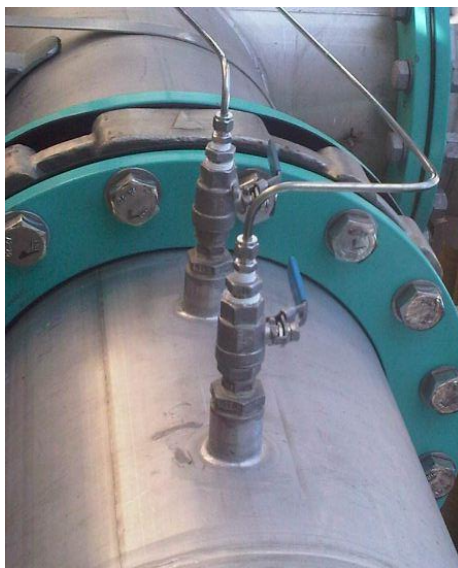
Figure 9 - Ball valve assembly
