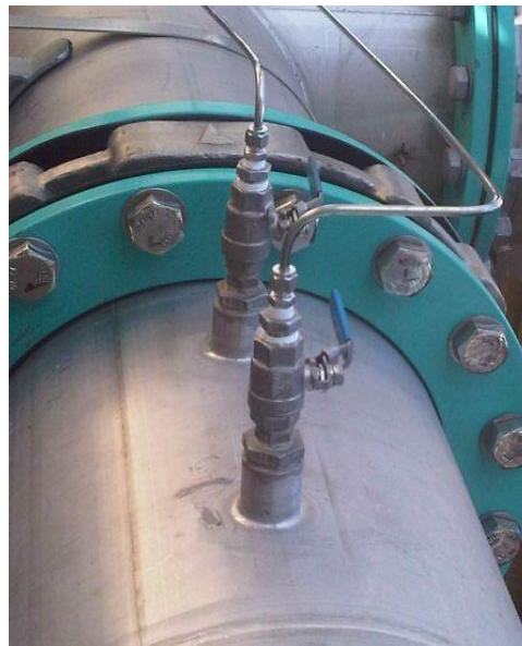
Figure 7 - Ball valve assembly
