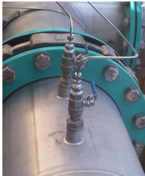
*Figure 5 - Ball valve assembly*
