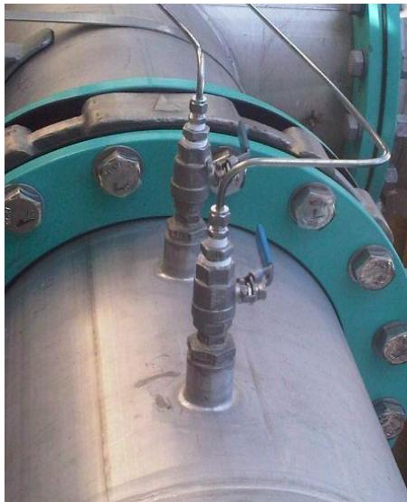
Figure 7 - Ball valve assembly
