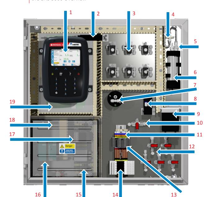
Figure 2 - BIOGAS 3000 internal components
