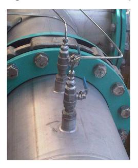
Figure 5 - Ball valve assembly
